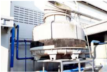
Power consumption reduction project in Faber-Castell's cooling tower in Indonesia Replacing the pump motor and installing a temperature regulator in the cooling tower at the Faber at the Faber-Castell factory in Indonesia meant that its average daily power consumption was halved from 0.50 MWh to 0.25 MWh. At the desired temperature, the pump motor shuts down and interrupts the electricity and water supply for cooling, so that resources are used more efficiently.
